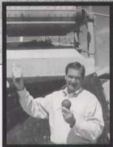
Top: Dykes Paving & Construction uses an Excel 3062 jaw plant to recycle concrete in a Blue Circle plant near Duluth, Ga. Inset: Jim Dykes with items recovered during recycling, including a bucket tooth and a cannonball.
