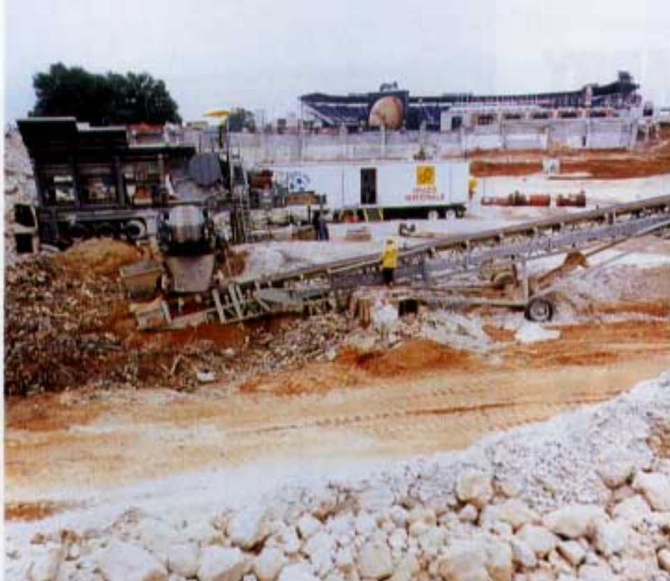
More than 120 tons of material was processed using the portable plant.
